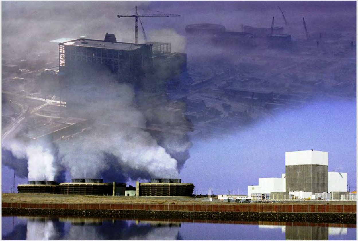
Top section: Columbia Generating Station under construction in the early 1980's and Bottom section: the way Columbia looks today. (Photo provided by Energy Northwest.)
