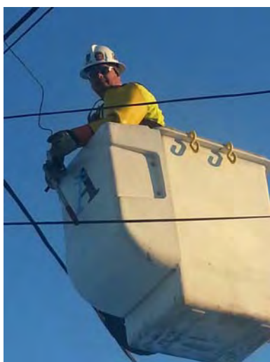
Michael Ferrier uses rubber glove handling to make repairs.
