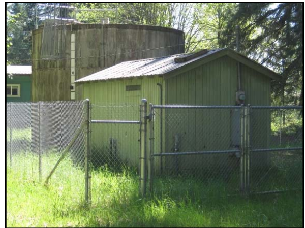
Arcadia Estates Well House and Reservoir in 2013
