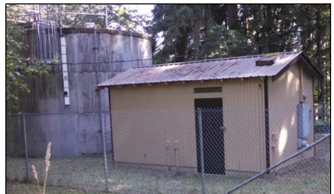
Arcadia Estates Well House and Reservoir in 2014
