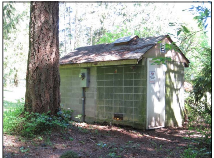
Bayshore Well House
