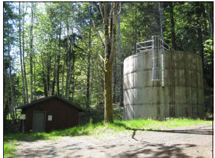
Canal Mutual Reservoir and Booster Station
