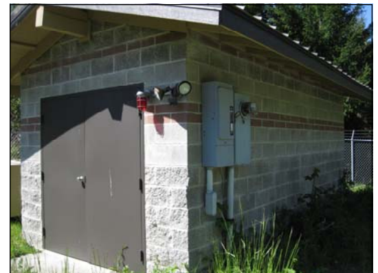
Reeder Well House
