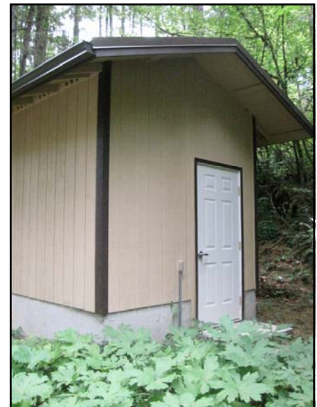
Hoodsport Suncrest Well House
