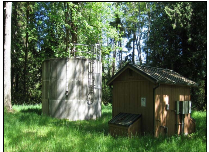
Pirate's Cove Well House and Reservoir
