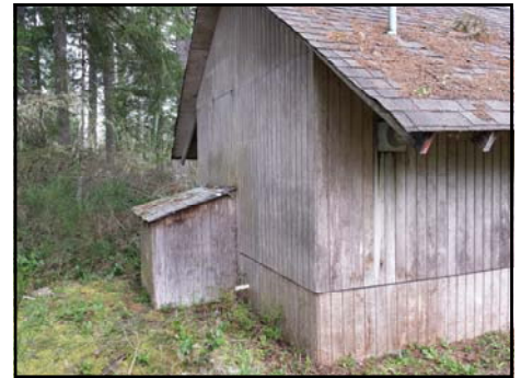
Ripplewood Well House
