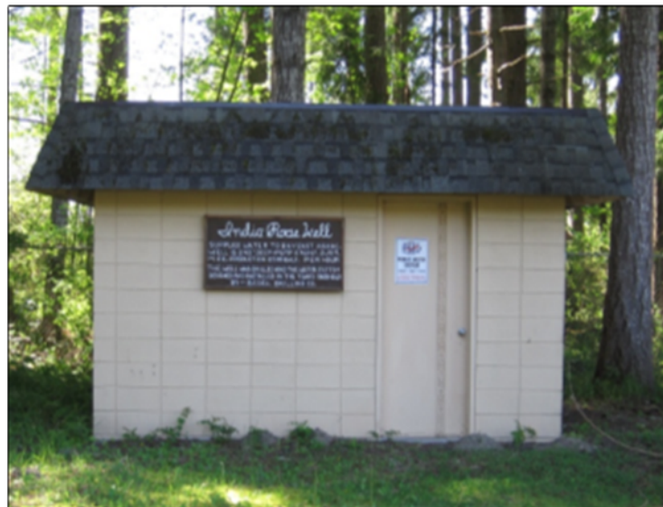
Bay East Well House
