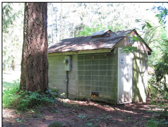
Bayshore Well House
