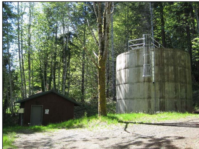
Reservoir and Booster Station
