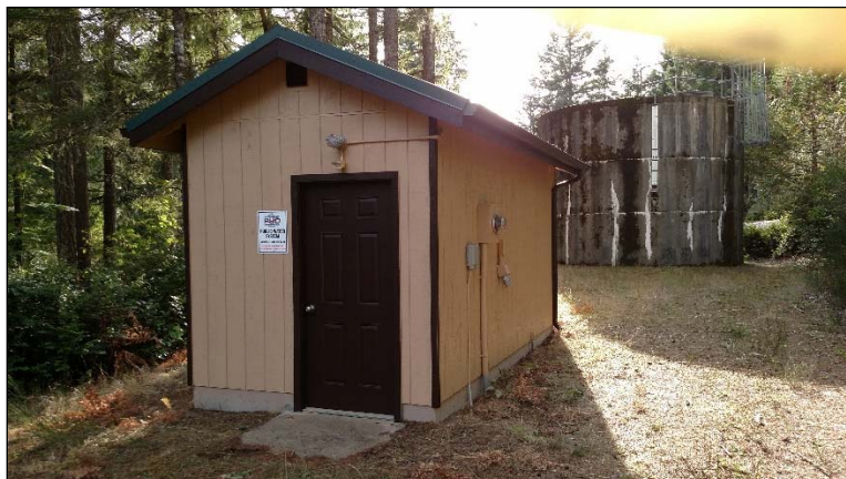
Booster Station, Reservoir and Well House
