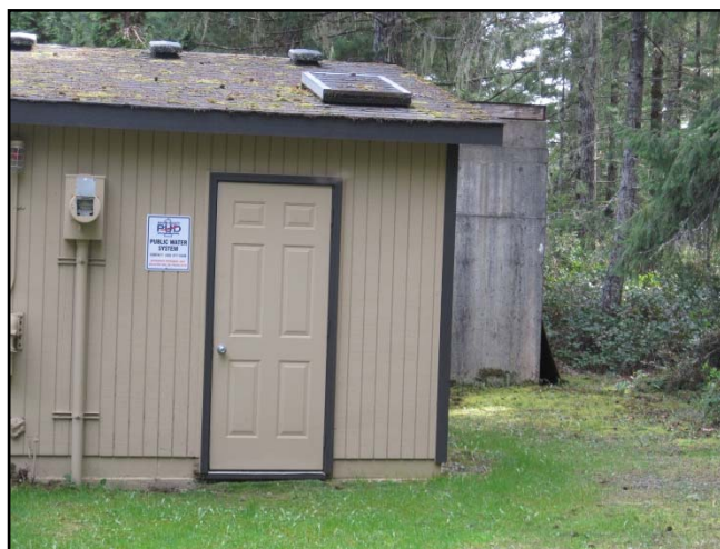
Well House and Reservoir
