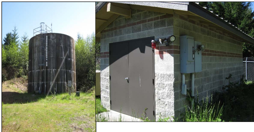
Reservoir and Reeder Well House
