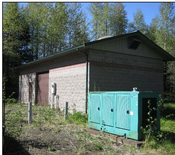
Pump House and Generator
