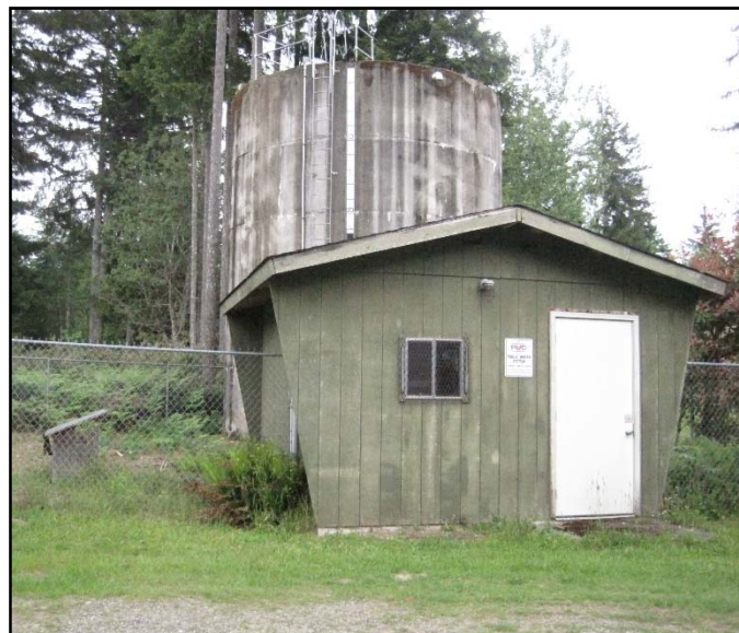
Pump House and Reservoir
