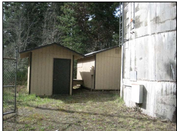
Booster Station and Reservoir
