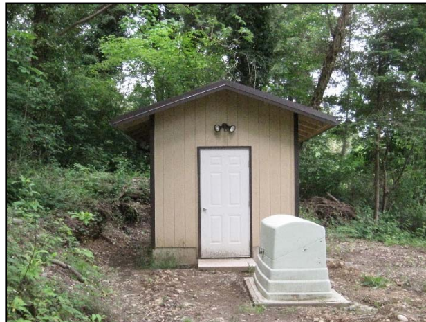
Pump House and Well 1
