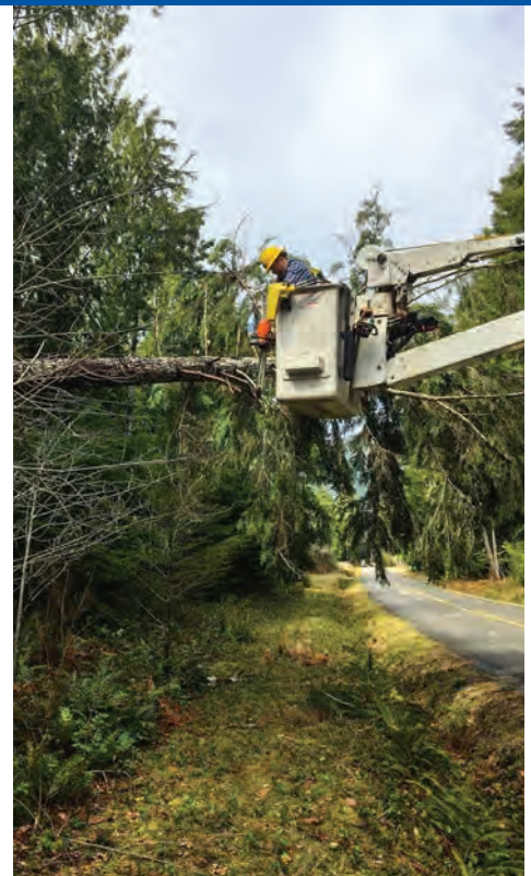
Lineman Tim Brown cutting trees out of line.
