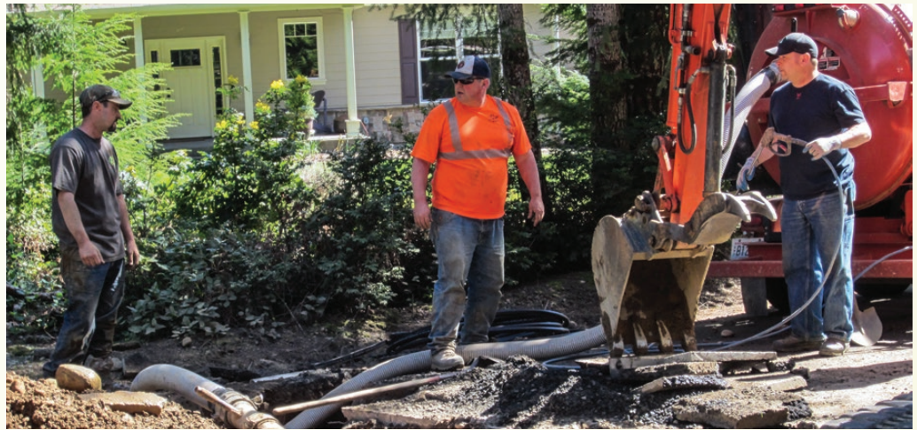
Replacing water mains in Alderbrook
