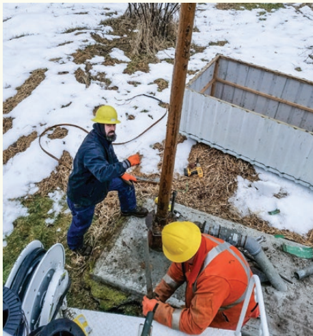
Emergency water pump replacement at Lake Arrowhead
