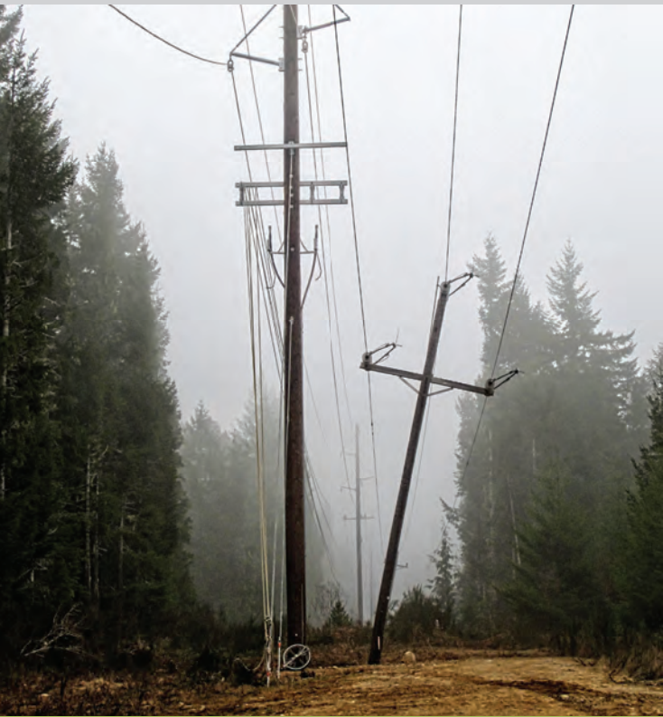
Old transmission poles (right) are replaced by new taller and stronger poles and wires.
