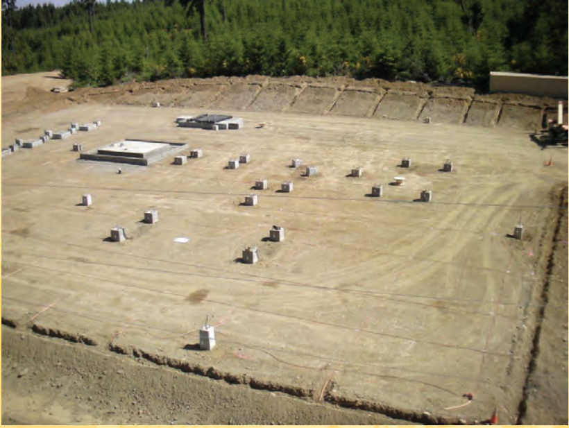
Concrete foundation has been completed for all incoming substation equipment and control buildings.
