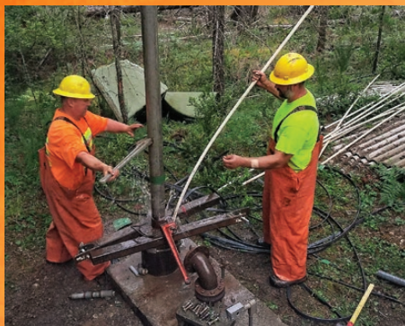
Well pump repair
