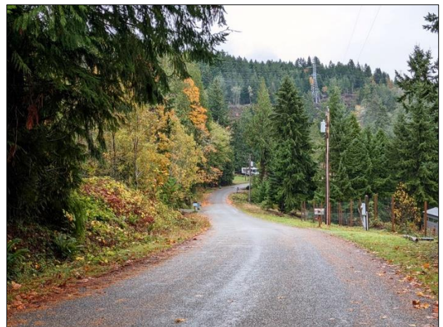
Figure A-6. View north to pole 3412 on Forest Drive in Triton.
