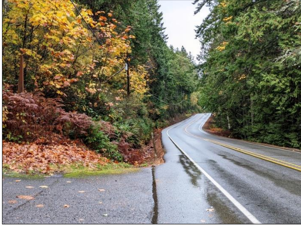
Figure A-30. View northeast to pole 3539 on U.S. 101.
