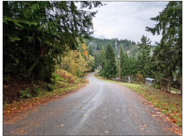
Figure A-5. View north to pole 3413 on Forest Drive in Triton.
