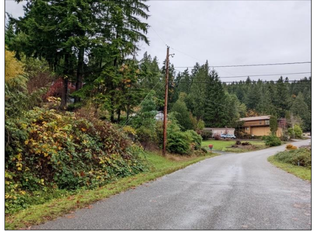
Figure A-10. View north to pole 3399 on Forest Drive in Triton.
