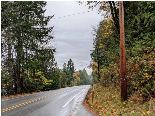
Figure A-14. View southwest of pole 3367 and 3339 on U.S. 101.
