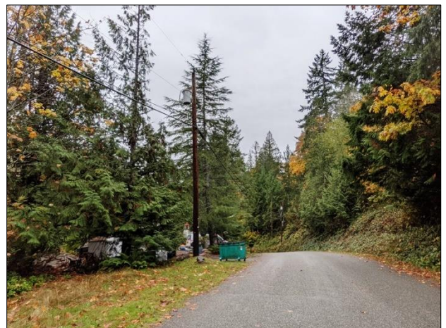
Figure A-12. View south to pole 3373 on Forest Drive in Triton.
