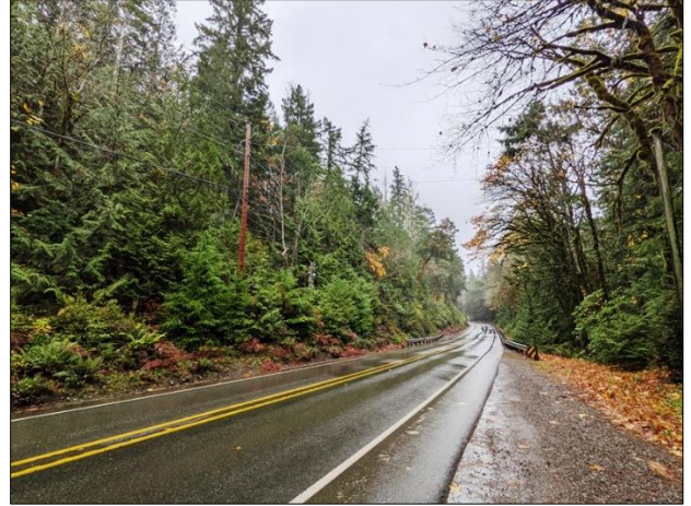
Figure A-33. View southwest to pole 5211 on U.S. 101.
