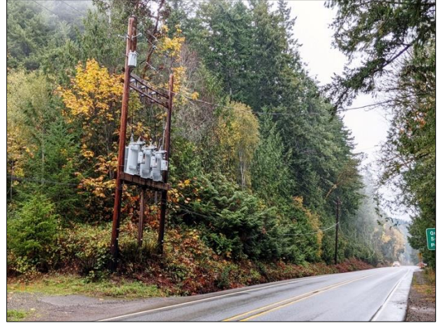
Figure A-15. View northwest to poles 3342, 3343, and 3345 on U.S. 101.
