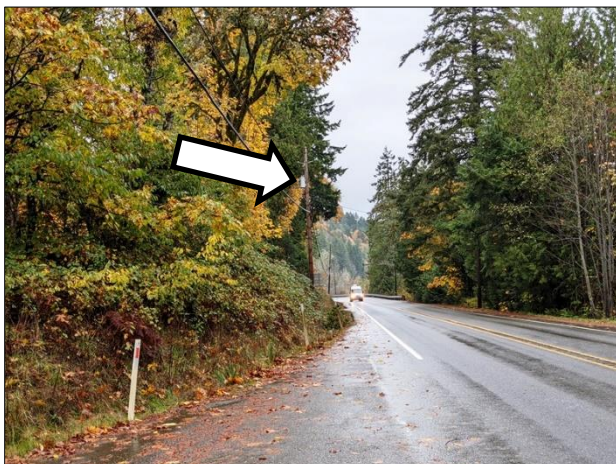
Figure A-15. View northeast of pole 3362 on U.S. 101.
