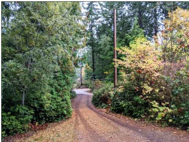
Figure A-25. View south to pole 3489 on unnamed road in Triton Head.
