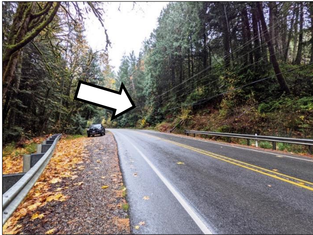
Figure A-31. View southwest to pole 3555 on U.S. 101.
