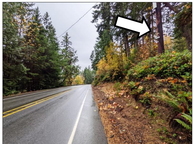
Figure A-29. View southwest of pole 3541 on U.S. 101.
