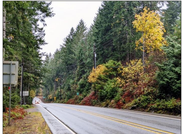
Figure A-16. View southwest to poles 3446, 3450, and 3454 on U.S. 101.
