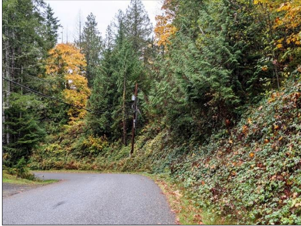
Figure A-13. View southwest to pole 3372 on Forest Drive in Triton.
