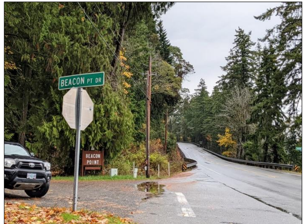
Figure A-28. View northeast to pole 3523 at N. Beacon Point Drive and U.S. 101.
