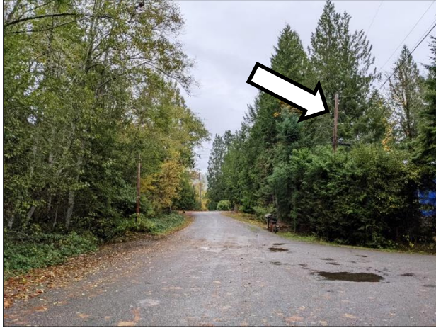
Figure A-1. View northeast to pole 3426 on Forest Drive in Triton.
