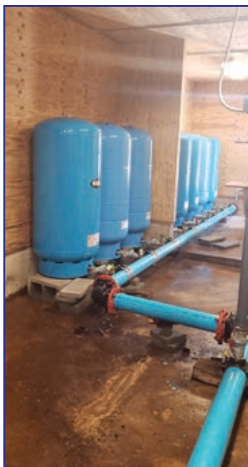
Air tanks installed at Rainbow Lake.
