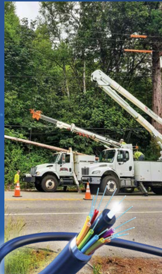
Magnum Power installing new pole line on Hwy 101
