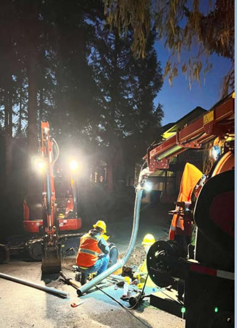
Early morning leak repair on Huckleberry Ct
