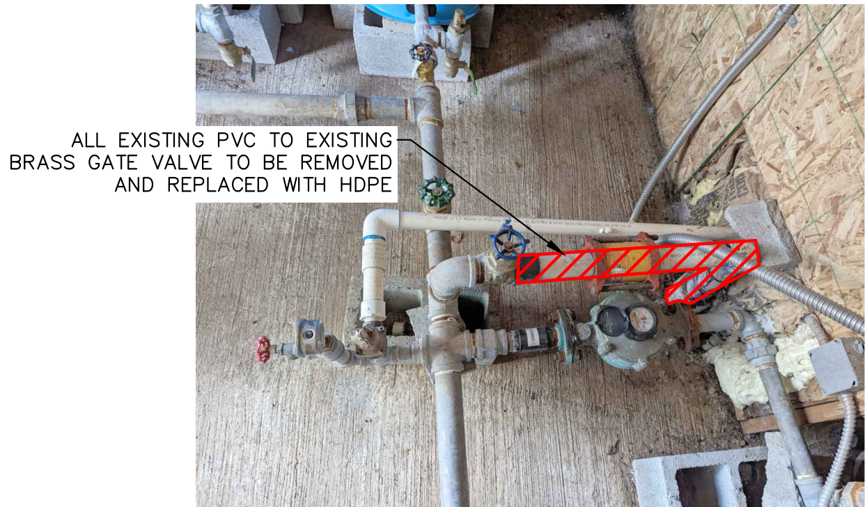
7 ABANDONMENT AND FINAL CONNECTION DETAIL (PAID AS SECOND CONNECTION) D.02 SCALE: N.T.S.
