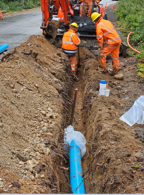
Installing new water line on E Westwood Ln W
