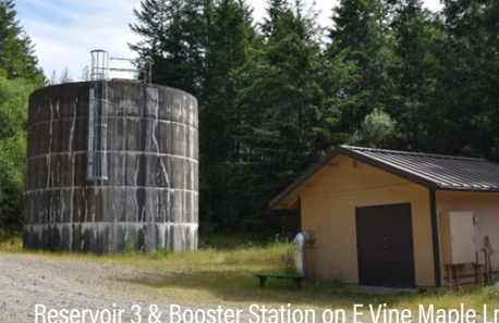
Reservoir 3 & Booster Station on E Vine Maple Ln
