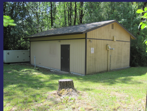
Booster Station & Backup Generator
