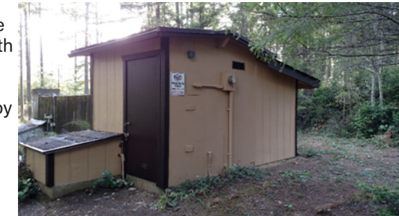
Well and Pump House
