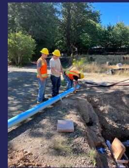
Installing main on E Tacoma St
