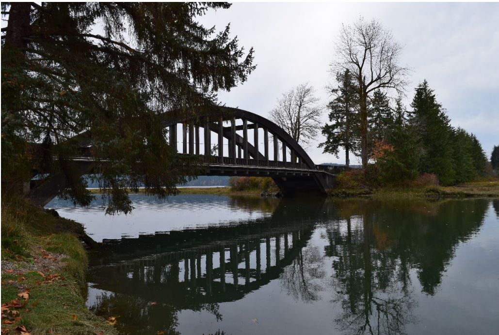
HAMMA HAMMA BRIDGE on US HWY 101, LILLIWAUP, WA
