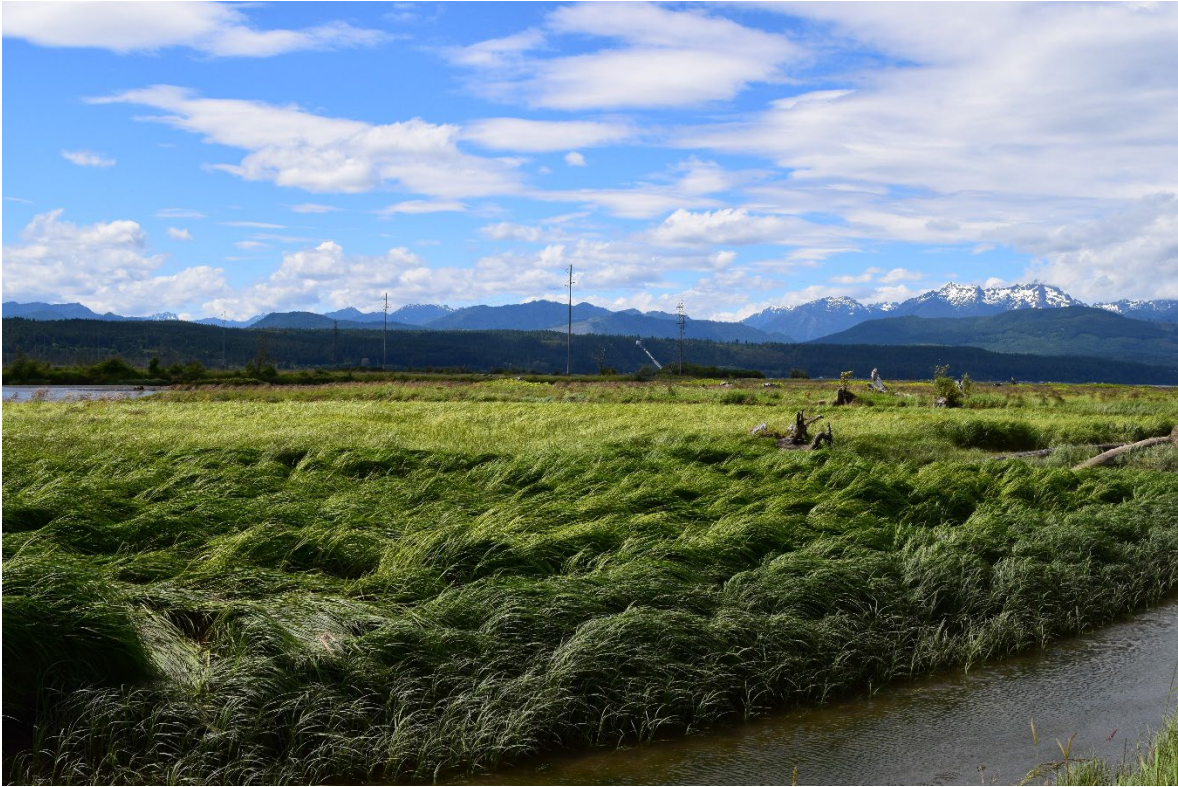
TRANSMISSION LINE ACROSS THE TIDEFLATS on HWY 106 to UNION, WA
