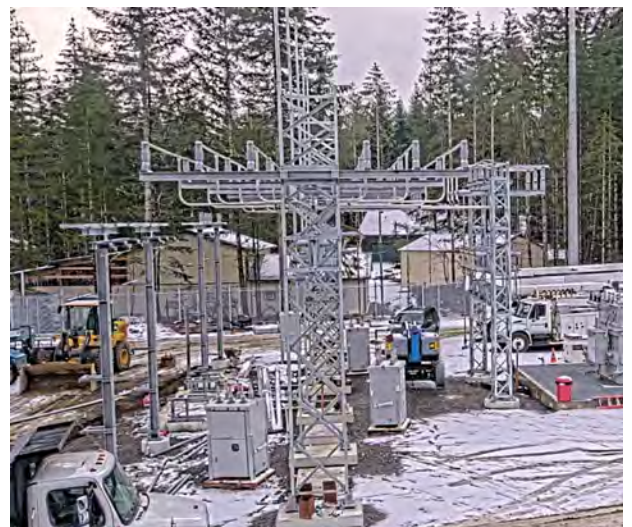
Steel structures erected at Manzanita Substation.
