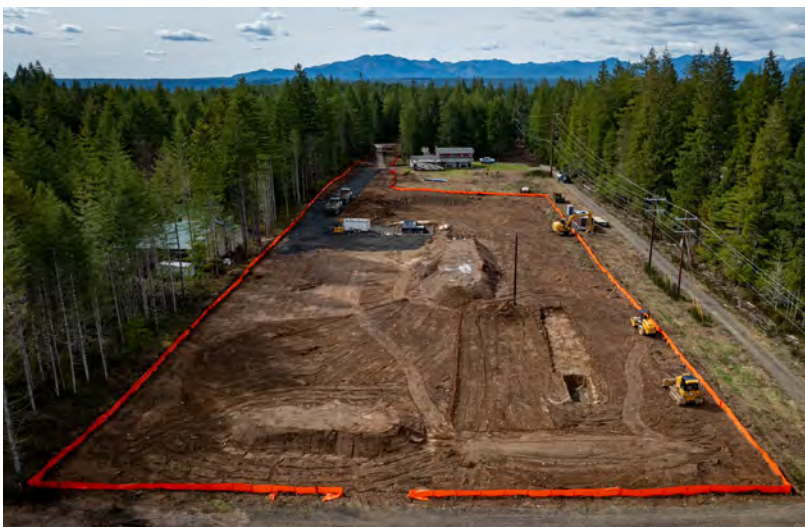
Site work in preparation for Manzanita Substation construction.
