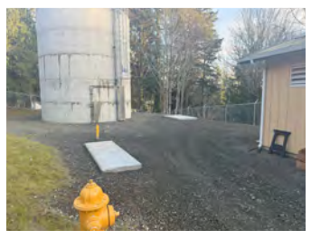
Concrete pads for Generator and Propane Tank
