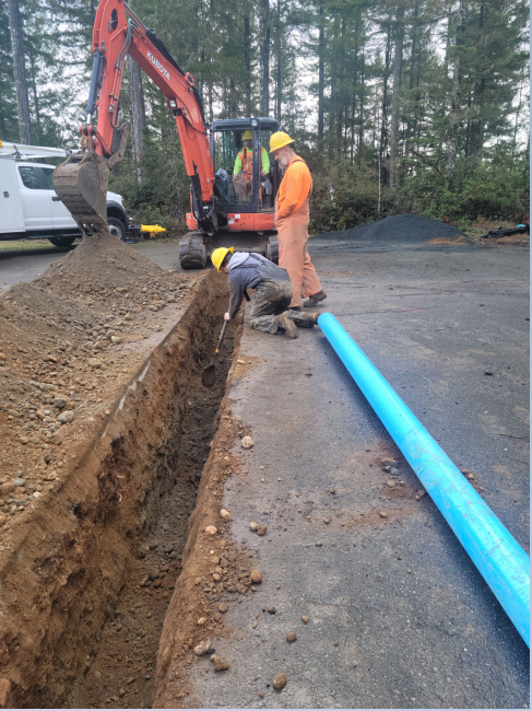
Installing new water line on E Dogwood Ct
