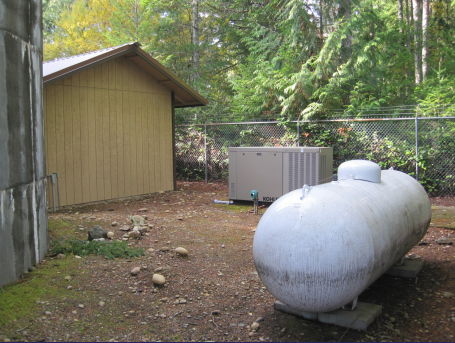
Backup Generator at the Booster Station
