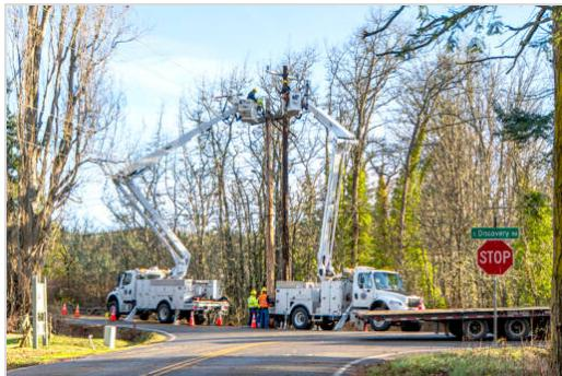
A crew from the Mason County PUD, in support of the Jefferson County PUD, works to replace a power pole and reconnect the power lines after a tree fell onto the wires and damaged the pole at the corner of Discovery Road and Cape George Road, near the Discovery Bay Golf Course. Powerful winds on Tuesday and early Wednesday morning knocked out power across the Peninsula. The majority had been restored by Wednesday. (Steve Mullensky/for Peninsula Daily News)
