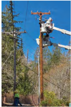
New Poles at Canal View
