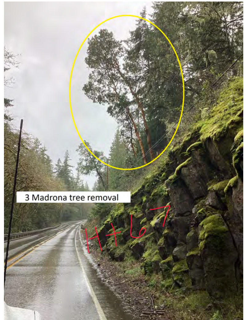
HT 67 Highway: SR101 Comments: 3 MADRONA TREE REMOVAL Latitude: 47.5807668025322 Longitude: -123.006317556002
