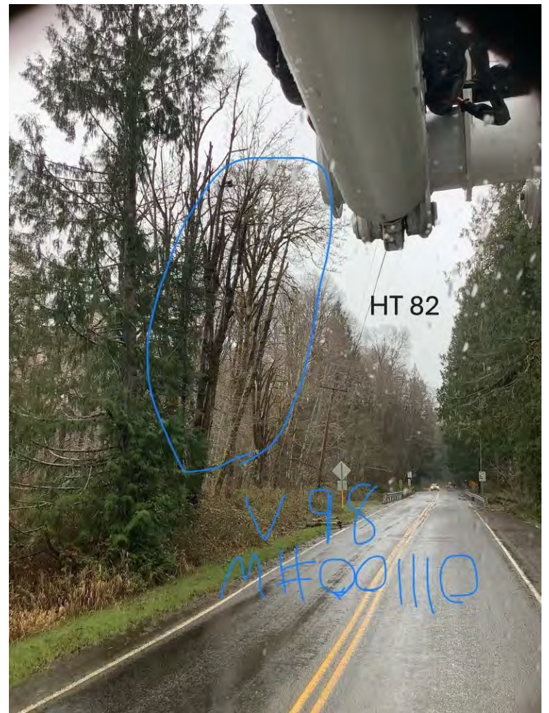
HT 82 Highway: W SKOKOMISH VALLEY RD Comments: 1 BIG ALDER REMOVAL Latitude: 47.31602895 Longitude: -123.2561455
