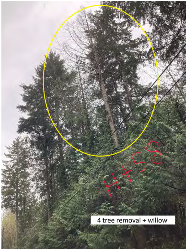
HT 58 Highway: SR101 Comments: 4 TREE REMOVAL + WILLOW Latitude: 47.63461872 Longitude: -122.9439368
