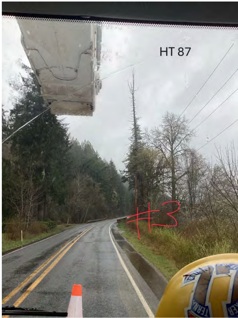
HT 87 Highway: SR106 Comments: 1 BIG FIR REMOVAL Latitude: 47.33093074 Longitude: -123.1169413
