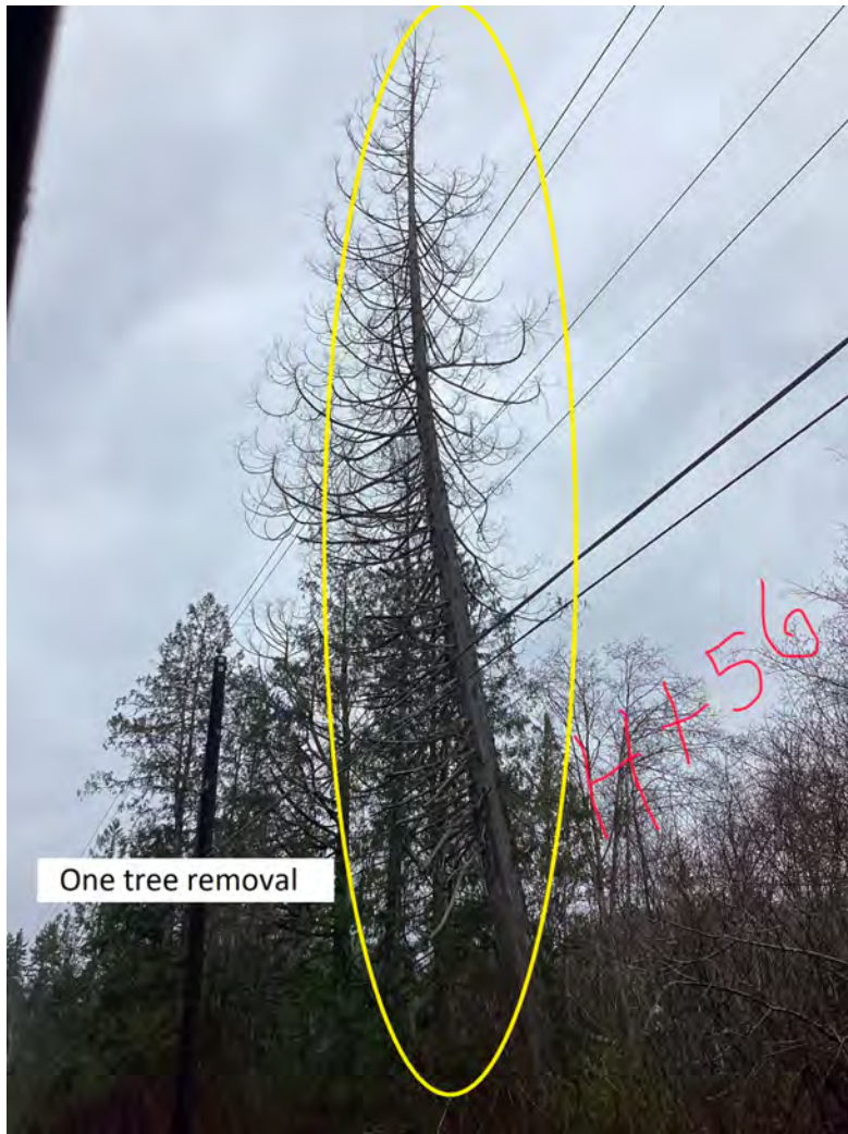
HT 56 Highway: SR101 Comments: 1 TREE REMOVAL Latitude: 47.63977547 Longitude: -122.9399742
