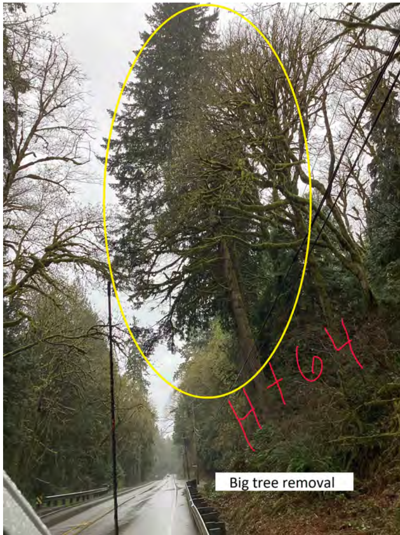
HT 64 Highway: SR101 Comments: BIG TREE REMOVAL Latitude: 47.5854842 Longitude: -123.0040663
