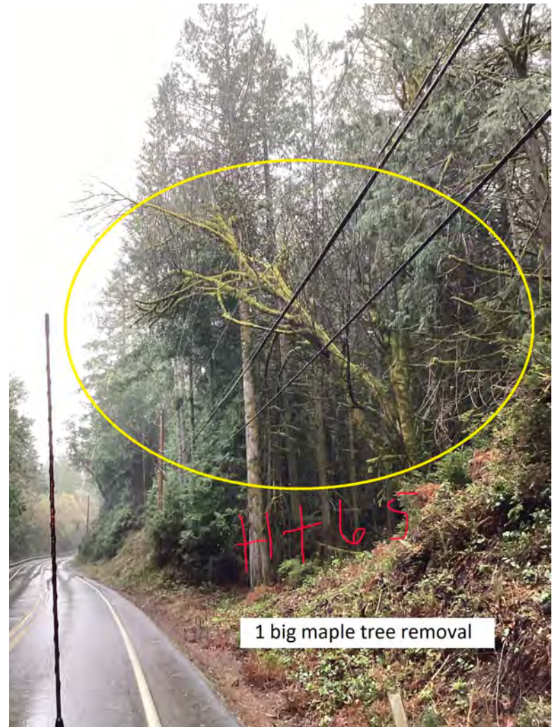
HT 65 Highway: SR101 Comments: 1 BIG MAPLE TREE REMOVAL Latitude: 47.58156463 Longitude: -123.0062099
