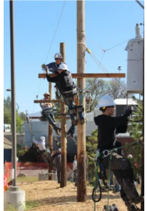
During Okanogan PUD's Industry Bootcamp, students use climbing gear to learn how to do typical tasks lineworkers perform.
