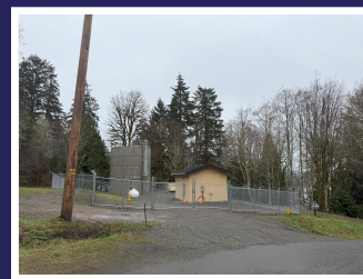
Reservoir and Booster Station Building
