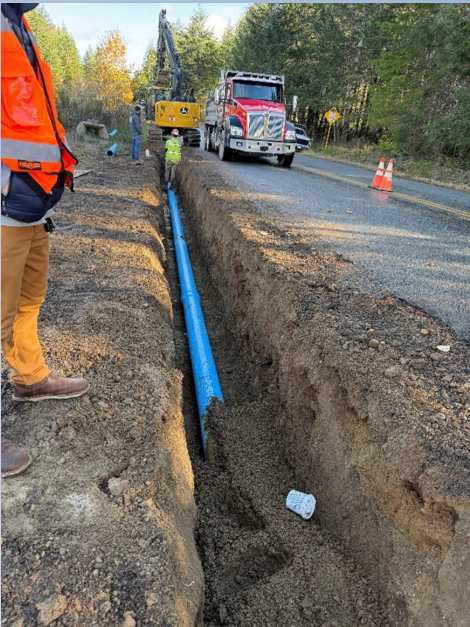
Contractor installing mainline on E Manzanita Dr
