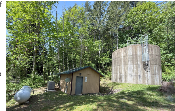
Canal Mutual Reservoir, Booster Station, and Backup Generator
