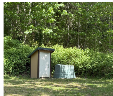
Chlorination room and well enclosure
