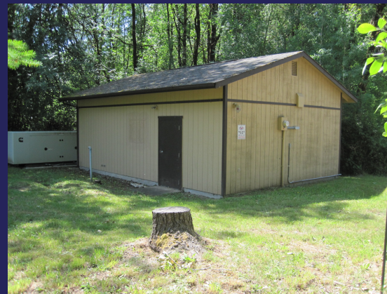
Booster Station & Backup Generator
