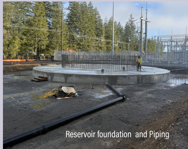
Fill lines being pressurized
