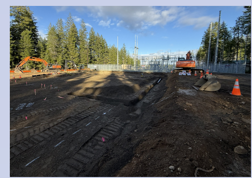
Site being prepped for Reservoirs
