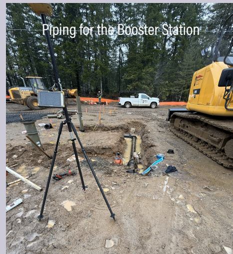
Fill lines being pressurized
