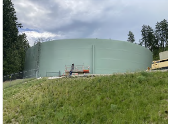
Photo courtesy of Vera Water and Power.
