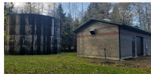
Reservoir and Booster Station
