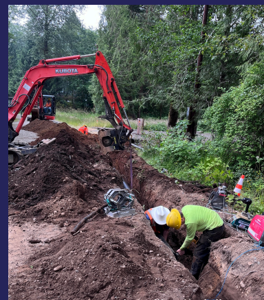
Water crew installing mainline
