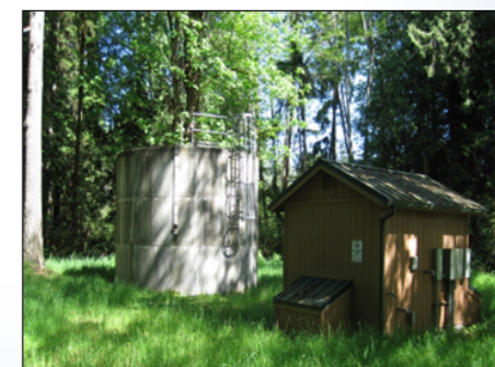
Well House and Reservoir
